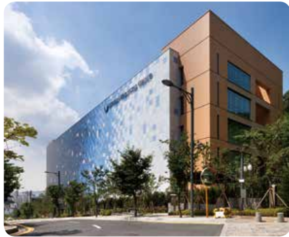
Shinhan Bank, Environment-friendly Green Building (Shinhan Data Center)
