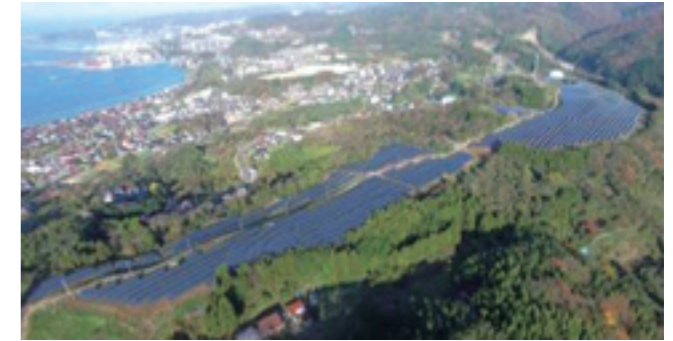
The 12MW solar power plant in Hamada in Shimane Prefecture Japan
